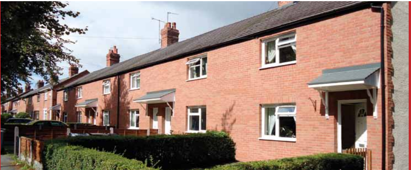
Terraced Housing Refurbishment, Middlewich, Cheshire | Brickshield
