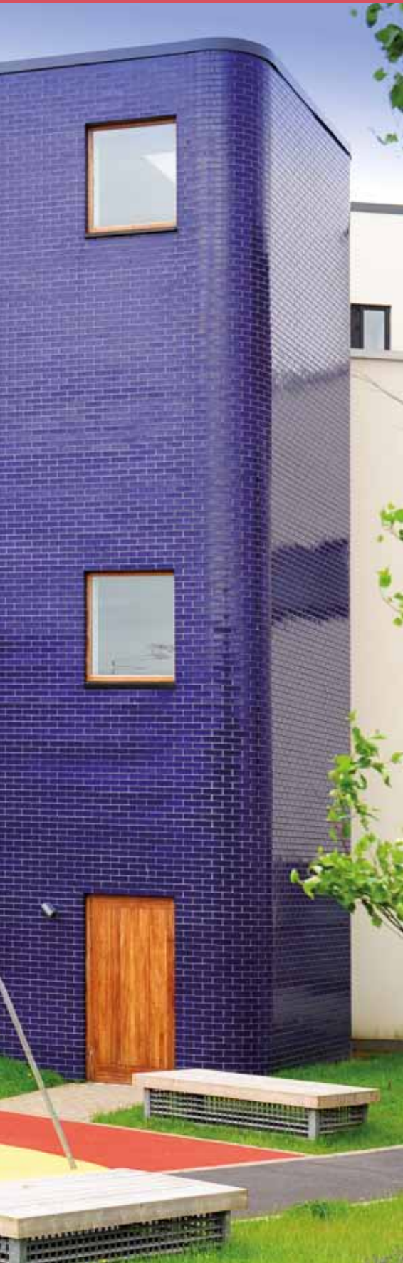
Civic Centre, Killorglin, Ireland | Blue Glazed Bricks
