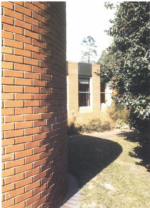
Figure 1 Faceting due to difference of arc and chord
