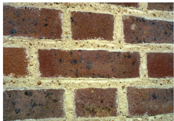
Characteristic appearance of Hydraulic Lime Mortar
