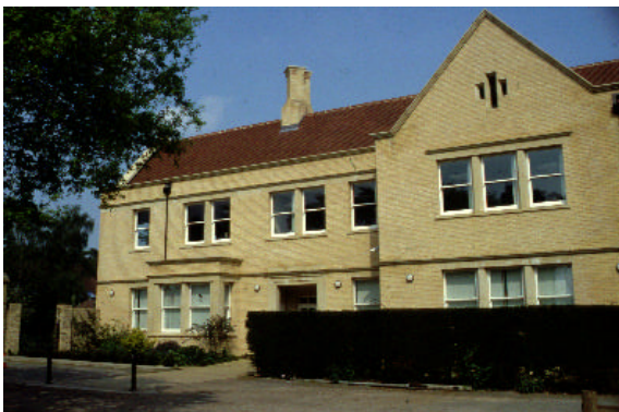
The new RSPB headquarters was constructed using an hydraulic blue lias lime mortar
